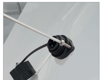
[Figure 15] Fasten the connector with two wood screws
